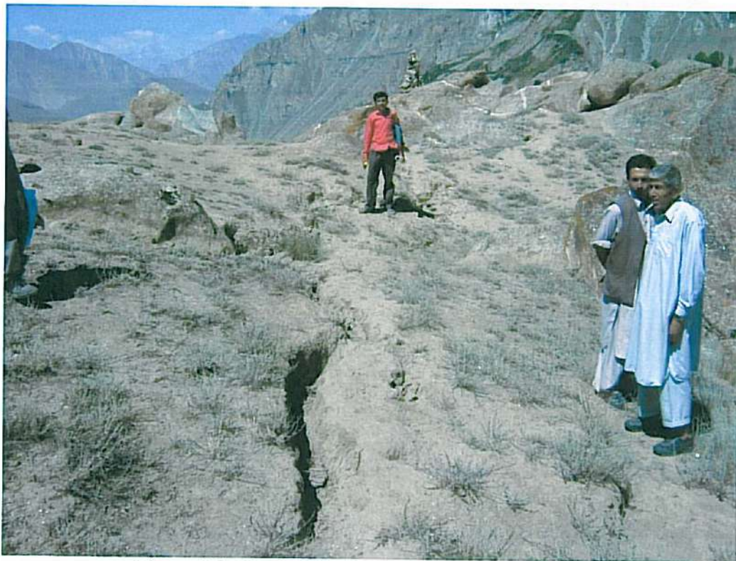
Figure 3.3: Crack widening at the left margin of upper slope
