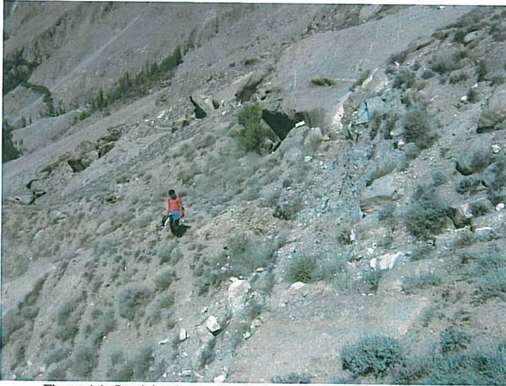
Figure 4.1: Semicircular crack with large displacements at backslope
